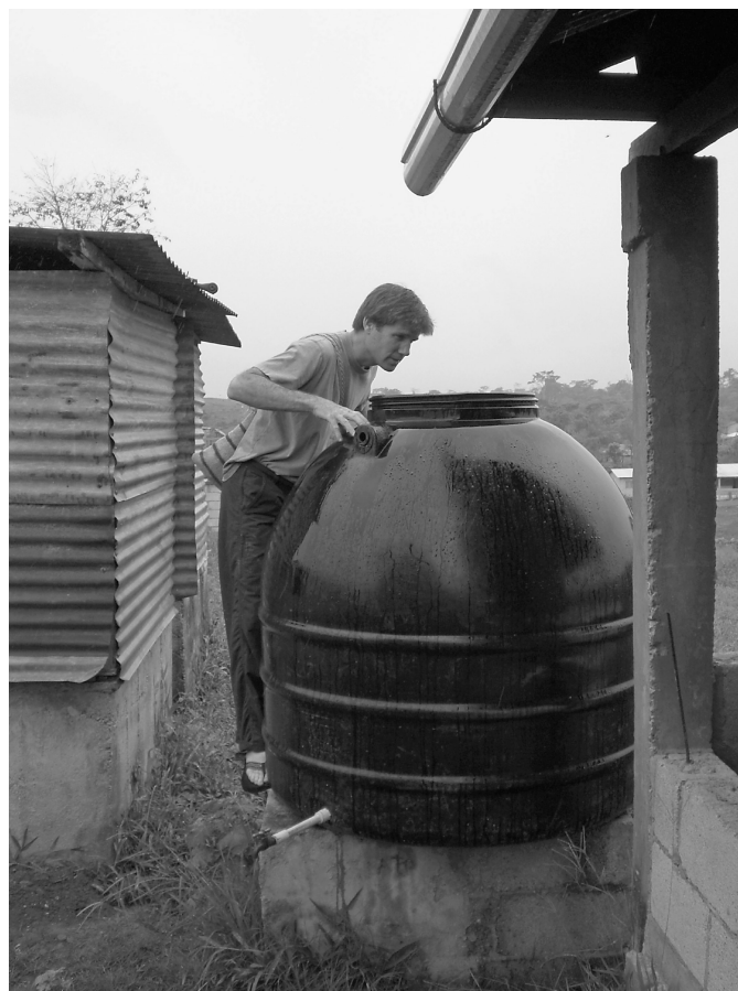
Figure 3. We installed rainwater catchment tanks to ensure a steady water supply to the school and health clinic during the dry season. San Lucas, Ixcán, Guatemala; June 2005.
